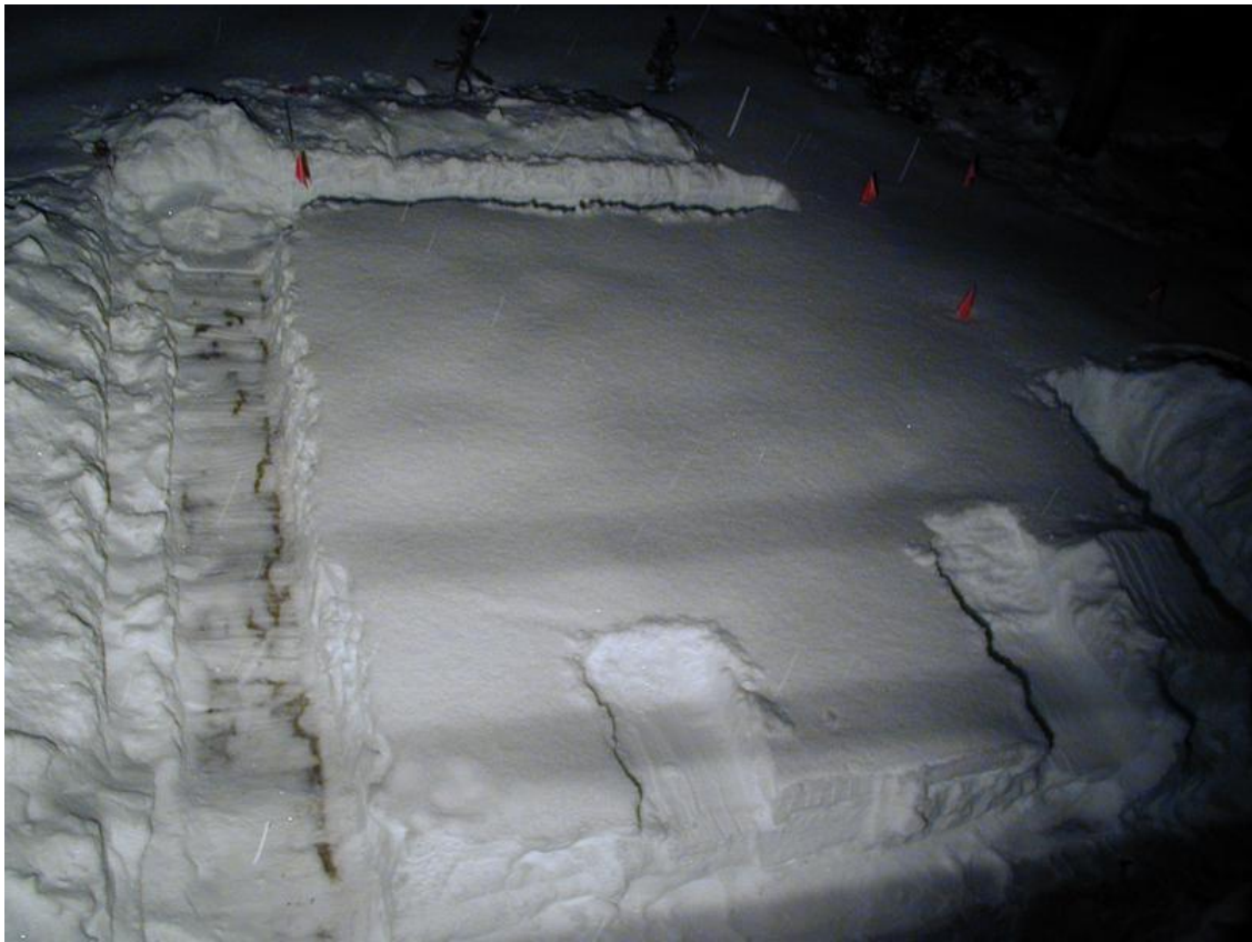
Figure 3. Dec. 13, 2002: Beginning of partial removal
